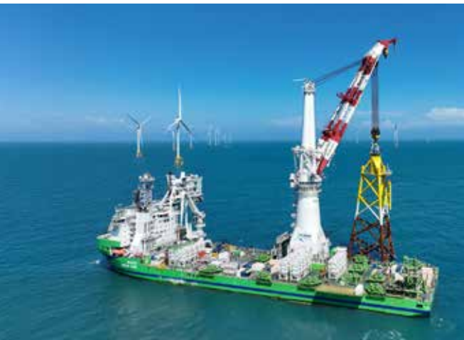
DEME • Green Jade at the Hai Long offshore wind farm, Taiwan
