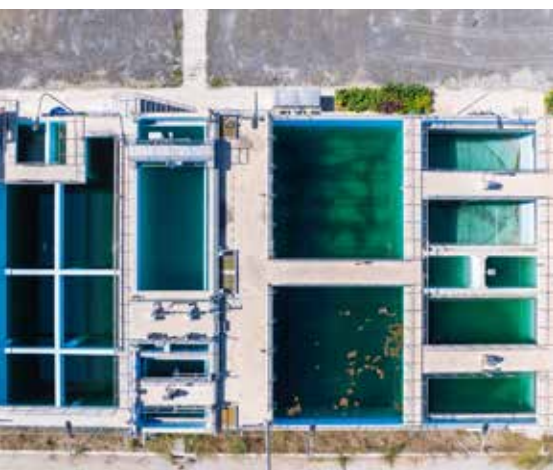
Deep C Holding • Waste water treatment at an industrial zone, Vietnam.
