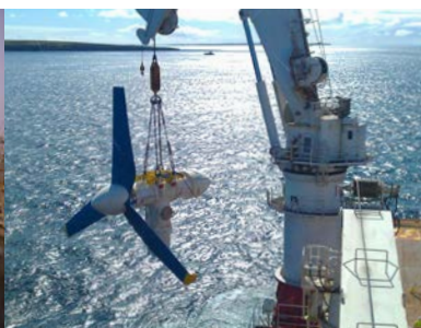
DEME - Installation of a tidal turbine
