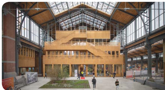
CFE Contracting - Gare Maritime - Brussels
