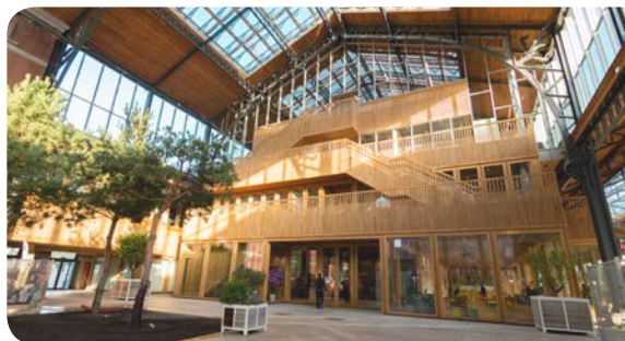
Extensa - Tour &amp; Taxis - Gare Maritime - Brussels
