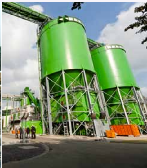
Max Green - Rodenhuize plant - Ghent
