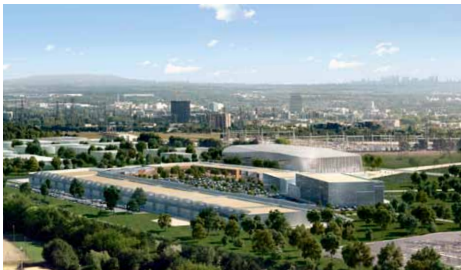
CFA - Aren'Ice and Aren'Park - Cergy-Pontoise ©
