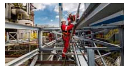
Scaffolding works at AVR (Rotterdam)
