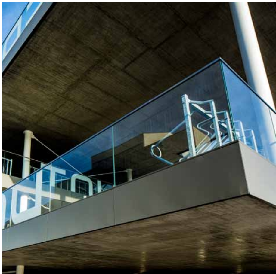
Fietsenstalling - Berchem station
