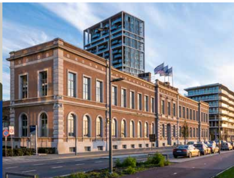
Bank Van Breda • Headquarters in Antwerp, Belgium
