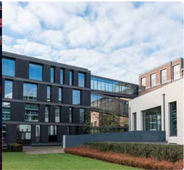
Bank Van Breda • Headquarters in Antwerp, Belgium
