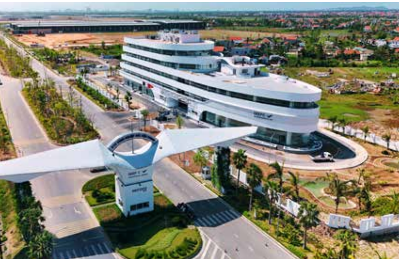
Deep C Holding • Service complex at DEEP C Quang Ninh, Vietnam
