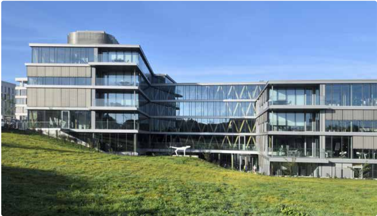
CFE • Wooden office building, Luxembourg
