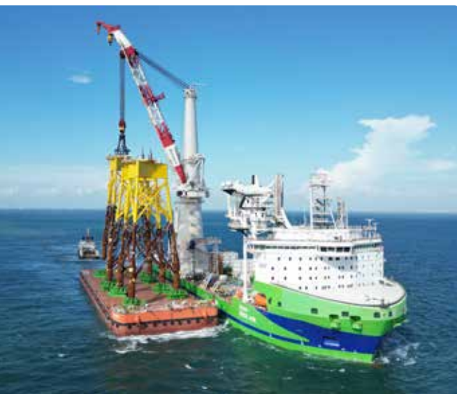
DEME • Offshore Energy, Zhong Neng
