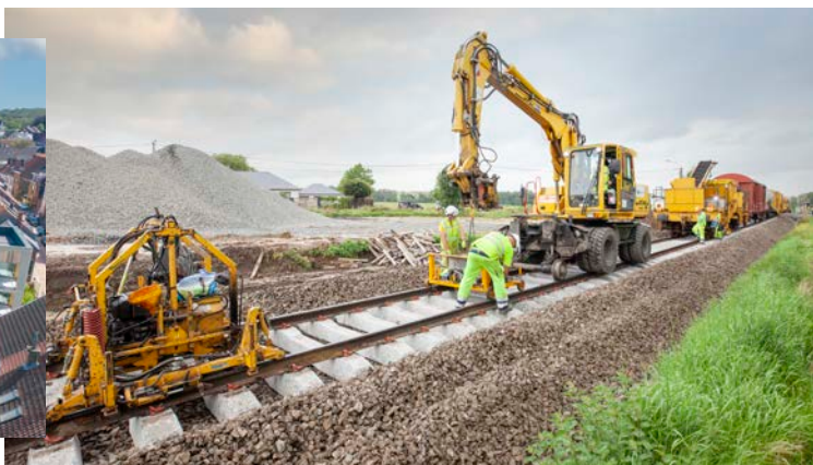
CFE &gt; Mobix, railway infrastructure works
